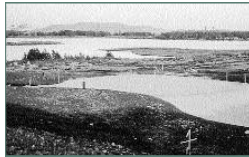
Harborside International as it appeared during construction.
