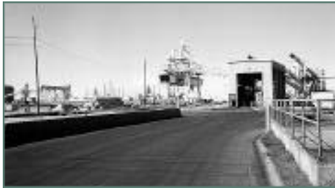
Stormwater filtration system and shiploader.
