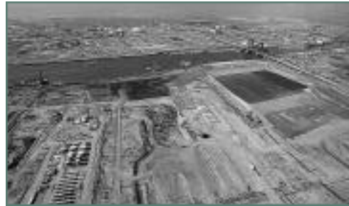
TCL site during remediation.
