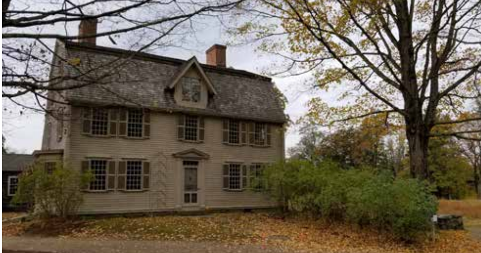
Figure 2. The Old Manse in 2018. View to the west.
