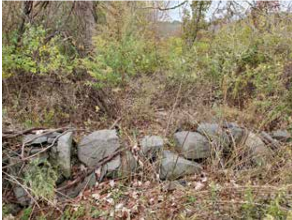
Figure 20. Southern wall section facing west.
