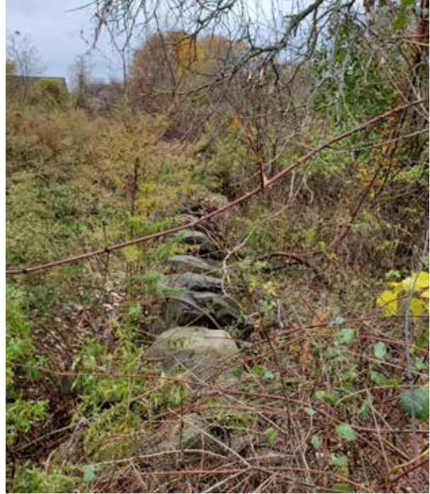
Figure 19. Southern wall section facing south
