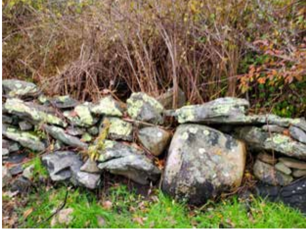
Figure 18. Middle wall section facing south.
