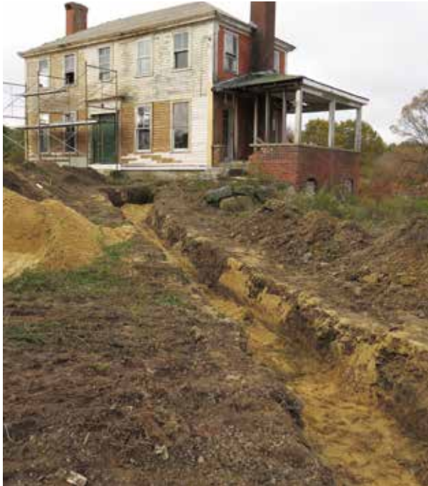
Figure 5. Utility trench, looking southwest towards the house.
