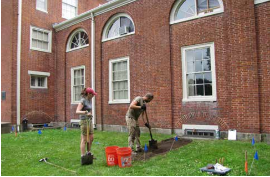
Figure 23. Starting excavation of EU205. Note that the unit abuts the window well of a cellar window with an arch in the brickwork above the window. The architects have interpreted the arch as evidence that this window and another cellar window to the east (left in the photograph) were once doorways. EU206, not yet excavated in this photograph, is located under the middle of the three large first floor windows.
