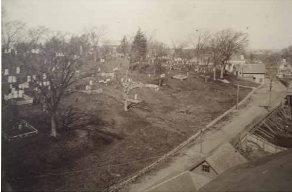
Figure 7. Photograph taken after the demolition of the stable buildings and school on School Street, looking north, before the area had been fully filled and graded.
