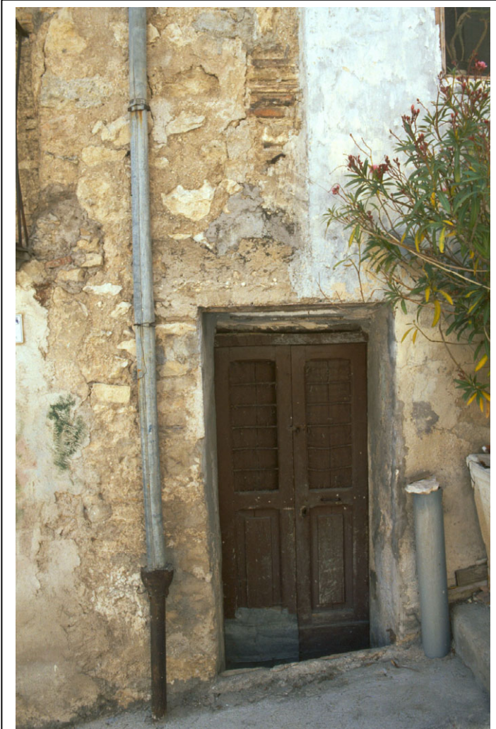
Figure 6.42: A doorway along a steep side street in eastern Lama, with an uncertain boundary of peeling stucco above, seemingly splitting its header in two.
