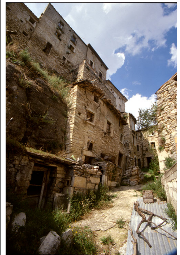
Figure 1.9: Lower Taranta Peligna, an upriver village near Lama and Colledimacine. This entire complex of buildings has been abandoned due to slow yet immense land slippage over time – a problem in various forms experienced throughout the valley.
