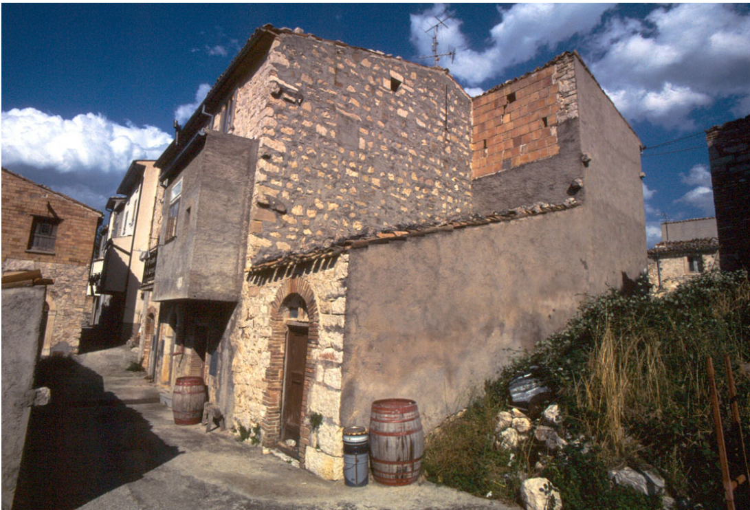
Figure 1.11: View of a side street in Colledimacine near its northwestern edge. Note the postwar repairs (from the patched wall at upper right, to the new story at center left), and recent extensions (perhaps for modern bathrooms). The vacant lot to the right is the site of a house destroyed during the Second World War that was never rebuilt.
