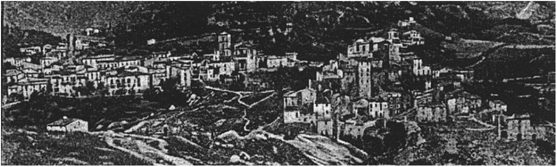
Figure 6.15: View of Lama in 1919, showing the split caused by frequent landslides, which have continued to the present; the portion at right, Old Lama, has now been almost completely carried away, while much of the portion at left has been repeatedly damaged or destroyed and then rebuilt (Del Pizzo, Enrico, La Linea 150).
