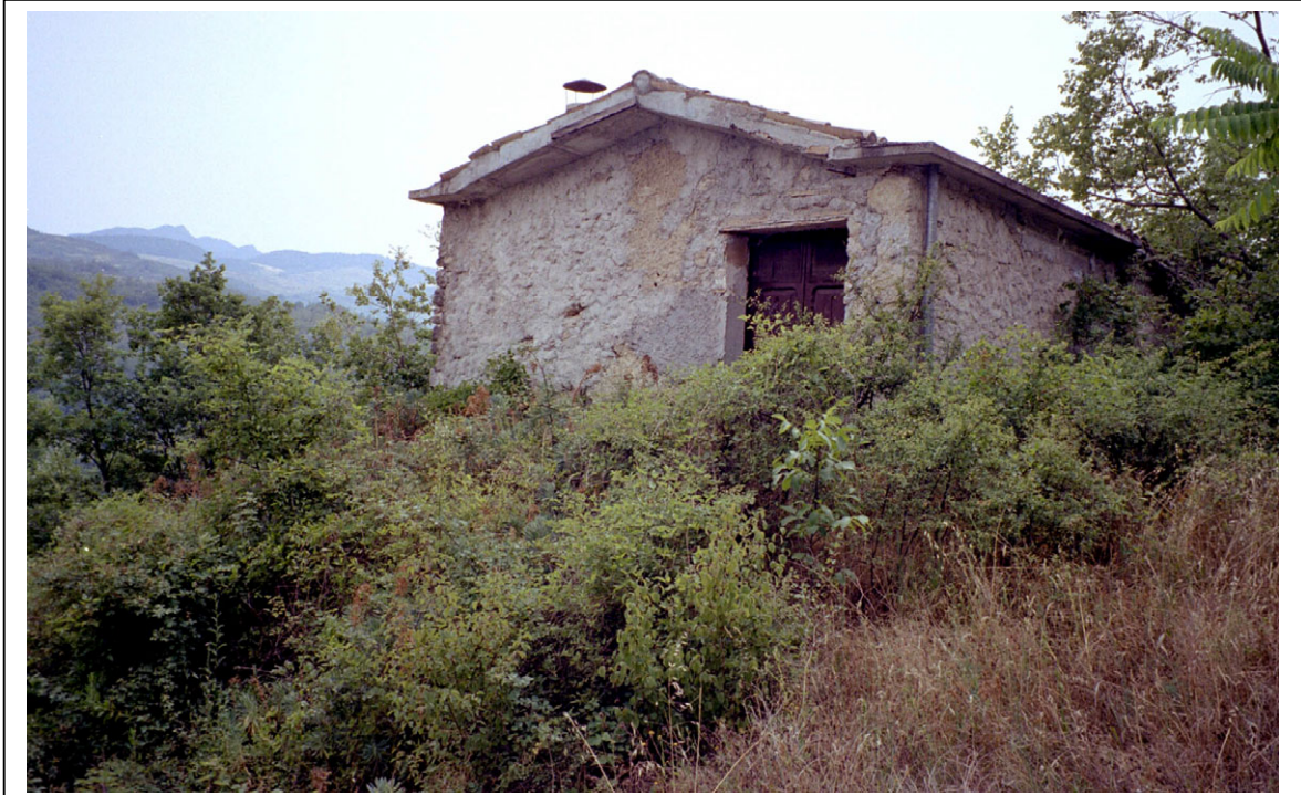
Figure 7.13: Abandoned house in Purgatorio at the bottom of the Aventino Valley.
