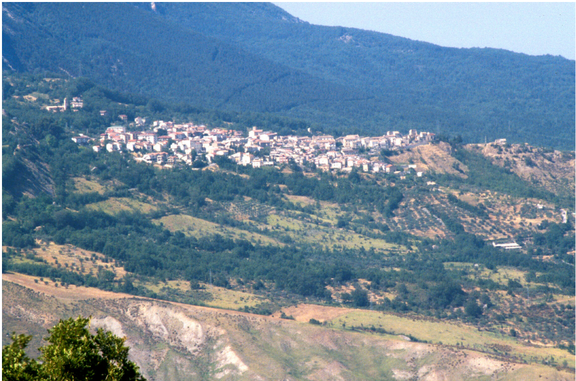
Figure 6.6: View of Lama from the Aventino Valley: note the convent at upper left, “Old Lama” at far right, the landslide area along the lower, right-hand edge of the village (beginning at the bare yellow patch and extending to the right and downhill all the way to the valley floor), and the scattered, mostly overgrown fields at bottom center.
