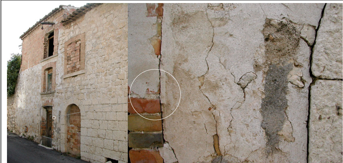
Figure 8.23: Two views of a building in Colledimacine: the close-up reveals what appears to be the rough boundary between two connected structures, lying somewhere between a stone and a brick doorway; the wide-angle image reveals the overall context.
