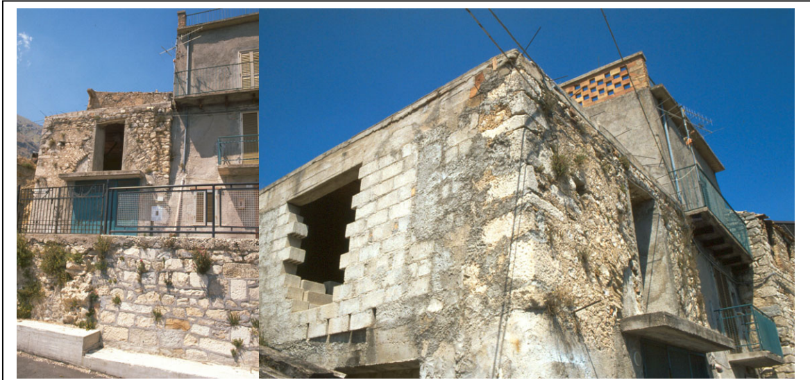
Figure 6.39: Two views of the same, long-unfinished building in eastern Lama, exhibiting a confusing mix of repairs to what appears to have been the remains of a war-damaged house, with a hodgepodge of various building materials, some recycled and some new.
