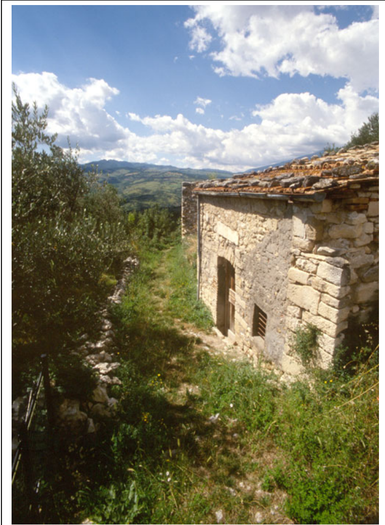
Figure 7.3: A building in Old Lama, once part of a house at the center of town, now a patched together rural outbuilding along its distant periphery.
