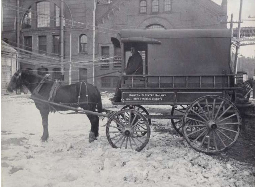
Figure 30. Photograph of a horse-drawn carriage operated by the BESRC to fix lines and conduits. From the 1989 WESR Inventory.
