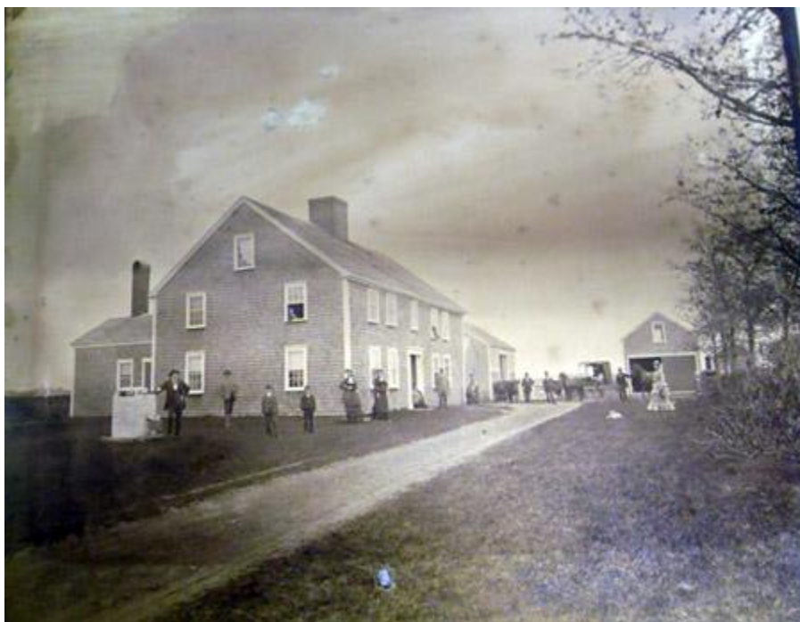
Figure 32: Wilbor house in c1876, unknown occasion. (LCHS)
