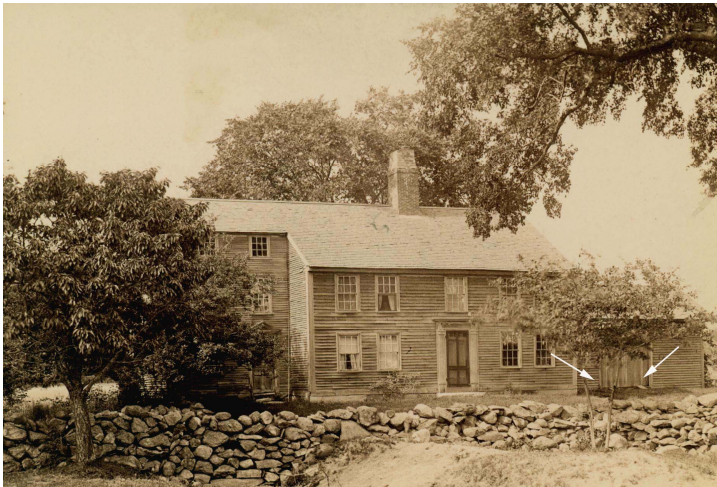
Figure 8: Historic photograph with arrows pointing to the “board ramps.”
